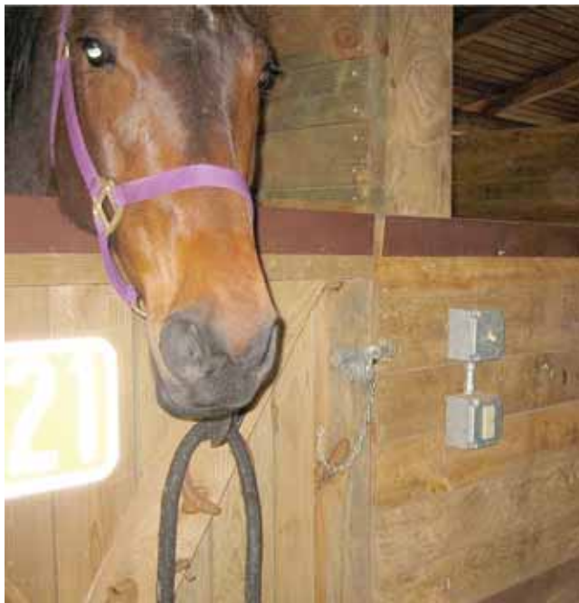
Fig. 1. Horse in a wooden structure with halter and lead rope at the ready. Other safety features include electrical components that are protected and in conduit, a reflective stall number, and an easy open latch. Photo courtesy of Tomas Gimenez.
