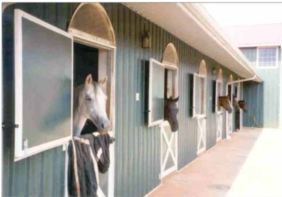
Fig. 7. Horses in this barn have egress through doors to the inside aisleway as well as to the outside. Dutch doors or paddocks off of each stall are highly recommended to allow responders access to animals even after smoke and fire are present. Photo courtesy of Dr. Tomas Gimenez.
