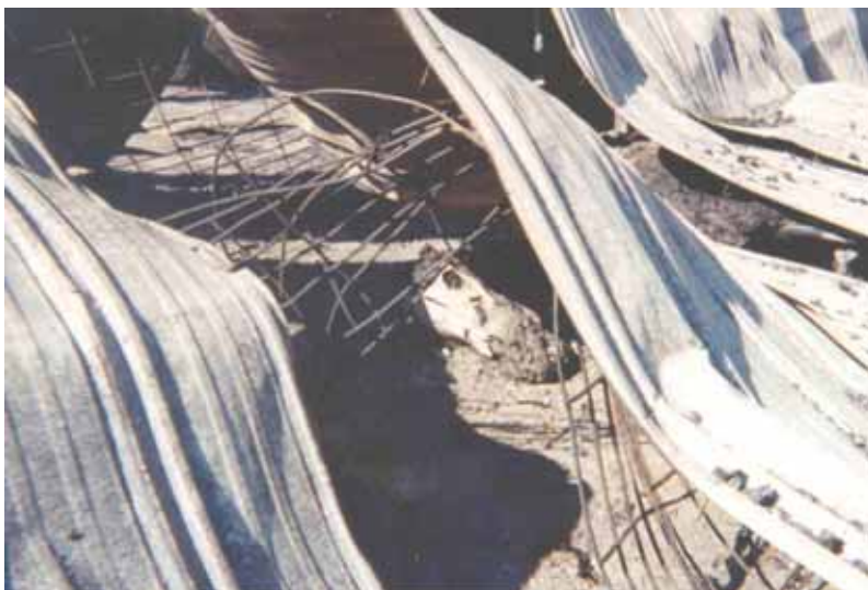
Fig. 8. The body of one horse in the Georgia fire is lying next to where the outside wall used to stand. Note hogwire and metal roofing. This facility was a total loss. Photo courtesy of Melinda Dennis.
