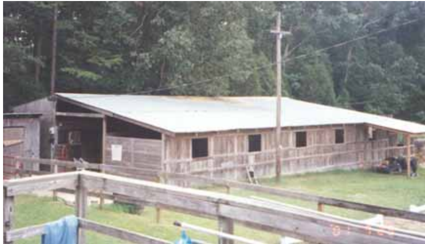
Fig. 13. Typical wooden horse barn. Photo courtesy of Tomas Gimenez.
