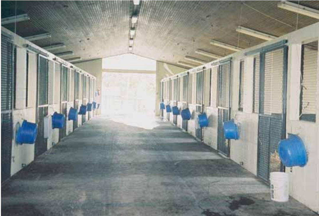
Fig. 10. The interior hallway of another well-constructed barn showing metal-rafter construction, hoses, doors to both the interior and exterior wall, and wide aiseways. Photo courtesy of Tomas Gimenez.
