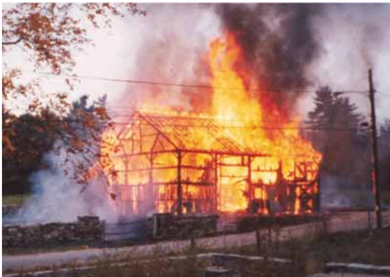
Fig. 4. A fully involved barn fire. Photo courtesy of Becky Kalagher.
