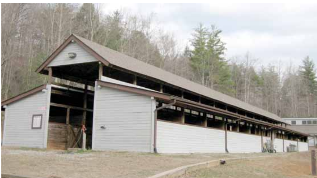
Fig. 16. Public horse barn built with fire safety in mind: open ventilation, frost-free hydrants, and 33 m of defensible space around the structure. Photo courtesy of Tomas Gimenez.
